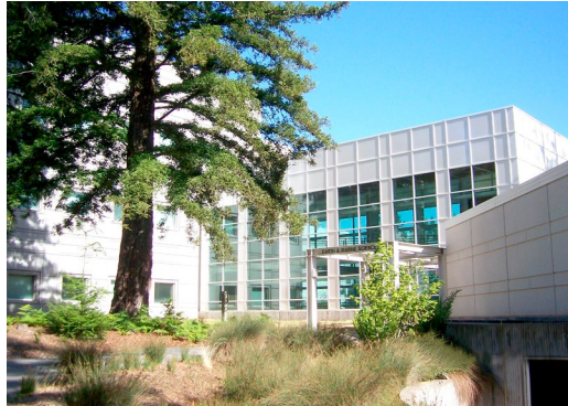
The Earth & Marine Sciences Building's high-use bathrooms were retrofitted with high-efficiency fixtures, resulting in substantial water savings. Image: Patrick Testoni.
